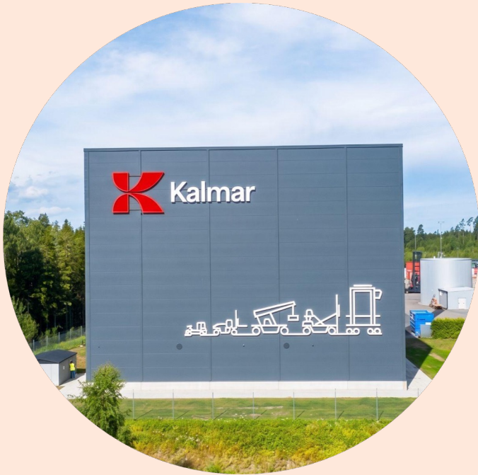
Industry-first fully automated Test Centre opened in Ljungby, Sweden
